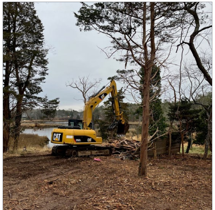
Demolishing a derelict boathouse on the restored property at Henson's Cove.
