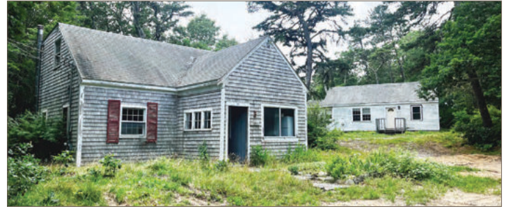
Two cottages slated for demolition.
