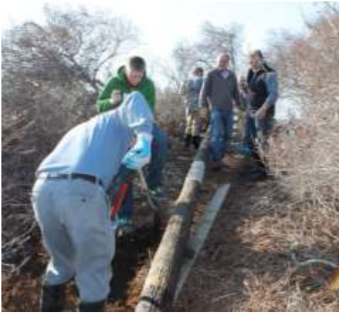
Hoisting pole up hillside
