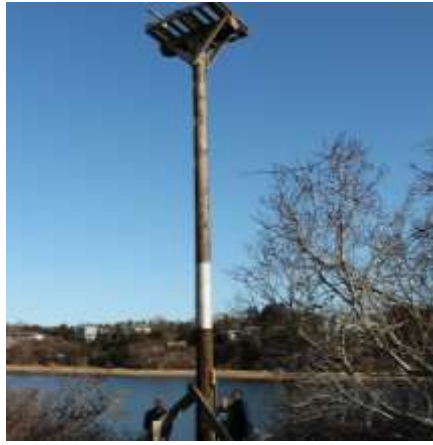
Stabilizing pole once up
